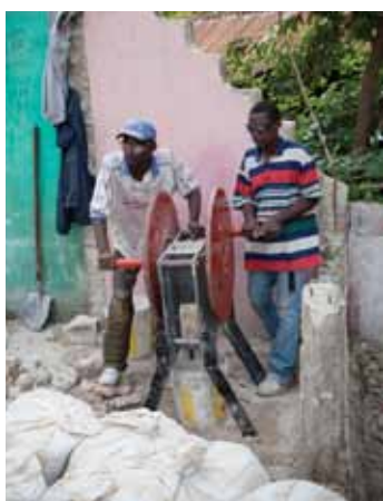
Porky (left) and Elizé (right) crush rubble from the demolished building they are standing in. They are making aggregate that will be used in concrete mix for new buildings.
